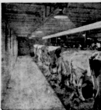
The above picture illustrates lighting outlets at 12-foot intervals on the center line of the litter alley and every 20 feet on the center line of the feed alley.
