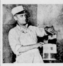
In removing this paint brush from a can of paint, it is always best to scrape off any excess fluid to prevent dripping or streaking.
