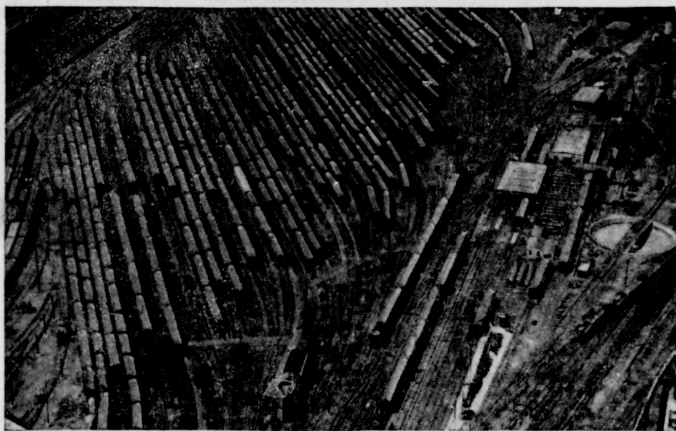
MARSHALLING YARD PACKS 'EM IN. Here is an aerial view of the Sunnyside yards of the Pennsylvania railroad at New York, the biggest railroad yards in the world. Even its great capacity was being taxed severely 24 hours before the scheduled national strike of three rail brotherhoods which didn't come off. Idle trains were being parked there in expectation of a complete stoppage of rail transportation. The strike, however, was delayed for eight days when President Truman seized the railroads in the name of the federal government and ordered the army to operate them. Leaders of the three unions—engineers, firemen and switchmen—obeyed a restraining order to postpone the strike. They remembered what had happened to John L. Lewis for ignoring the same kind of court order.
