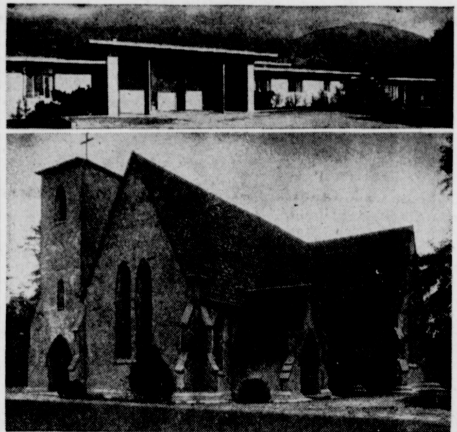
The old and new in rammed earth houses. Top panel shows modern structure at Claremont, Calif. Bottom shows church at Sumter, S. C., which has stood through more than a century and weathered several hurricanes and an earthquake.
