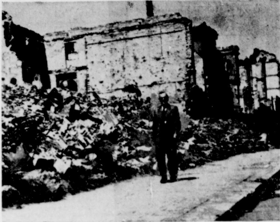
In midst of battered ruins of Munich, symbolic of shattered dreams of Nazism, former bund leader, Fritz Kuhn, walks streets in search of job. Deported to Reich after the war, Kuhn has settled with his family in the Bavarian birthplace of national socialism.
