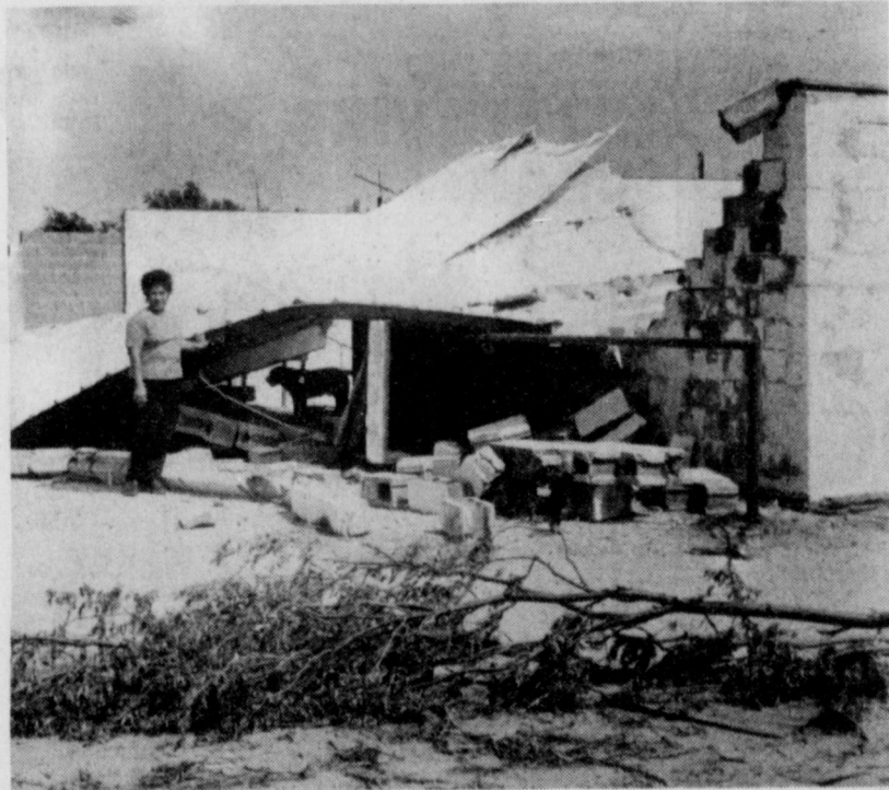
APARTMENTS DESTROYED---Ninfa Peacock stands beside one of the apartments in a farm labor housing complex that was destroyed in the tornado Friday night. (Journal Photo)
