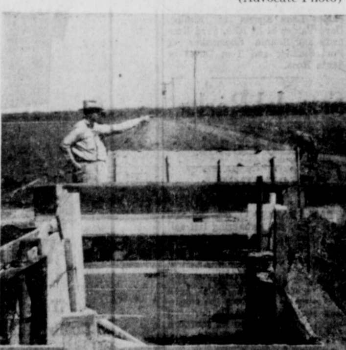
SCS ENGINEERS inspect a siphon structure under a roadway on a raised fill that has not yet been ditched, on the Langenegger project. (Advocate Photo)
