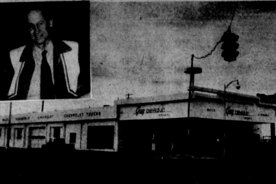
THE GUY CHEVROLET COMPANY'S re-modeled building and new service station which is re-opening with a week-long celebration starting Monday. Insert is Clyde Guy, owner (Advocate Photos)
