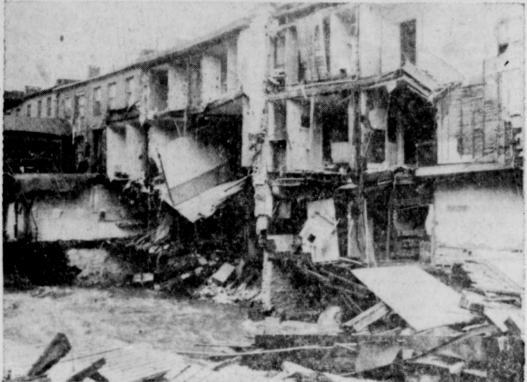
NORWALK—Overflowing Norwalk river left this devastation on main street. Walls of homes are ripped down in the city of 60,000. Ten inches of rain fell in 48 hours. (International Soundphoto)
