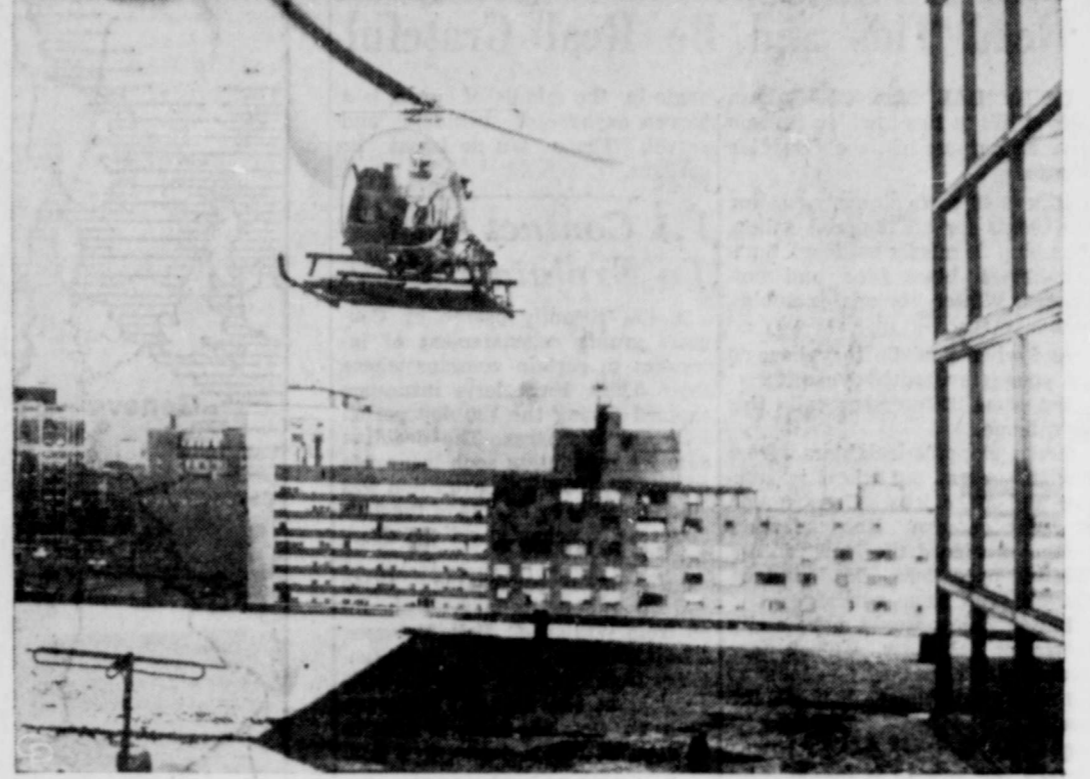
LASHED UNDER the helicopter is a plate of glass eight feet by seven, which is being delivered to a penthouse 21 stories up in Chicago. It wouldn't fit in the freight elevator, and balcony overhangs on the building made a block and tackle estimate to raise it hit $1,200. So Al Luke and his helicopter were hired for $800.
