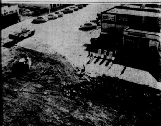
ARTH moving machines had the intersection of Main and First streets torn to pieces hursday as work on the urban project progressed on schedule. A dredging machine, rmed with a mammoth ball of iron, pounded the pavement into small chunks. Bulldozrs piled the debris up and trucks hauled it away. (Advocate Photo)
