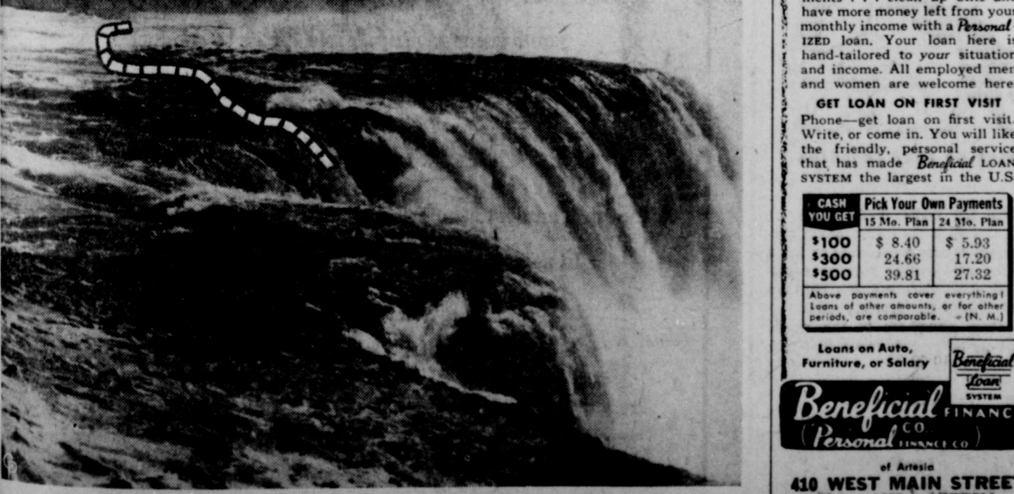
THE BROKEN WHITE LINE indicates the crack in Niagara Falls, N. Y., extending for about 80 feet back from the crestline of the American side of the Falls. The crevice is widening and engineers fear a new rockfall would take out a huge triangular portion of the crestline. (International Soundphoto)
