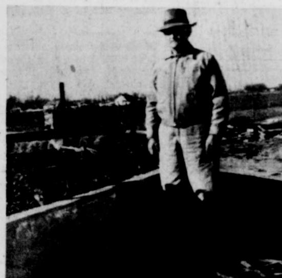
DISPOSAL plant superintendent G. T. Hearn checks another sometimes forgotten but highly important phase of the city's operation, located east of Artesia. The disposal plant requires a full-time attendant.
