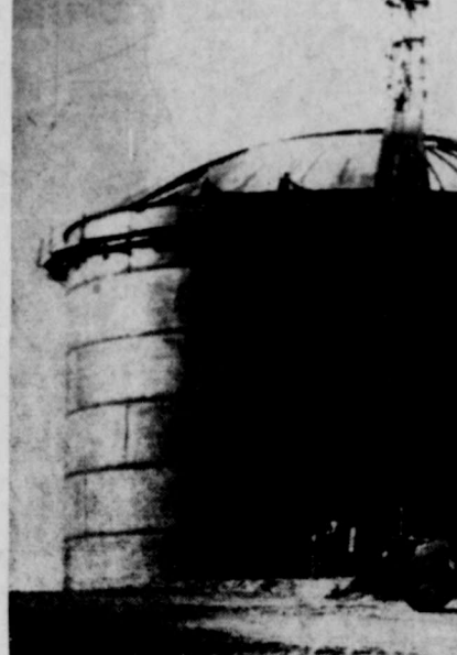
GIANT RESERVOIR west of Artesia nears completion. The reservoir will hold 2-million gallons of reserve water, giving Artesia better water pressure and reliable fire protection. Will be in operation by the beginning of the summer, after pipe has been laid and the reservoir painted. (Advocate Photo)
