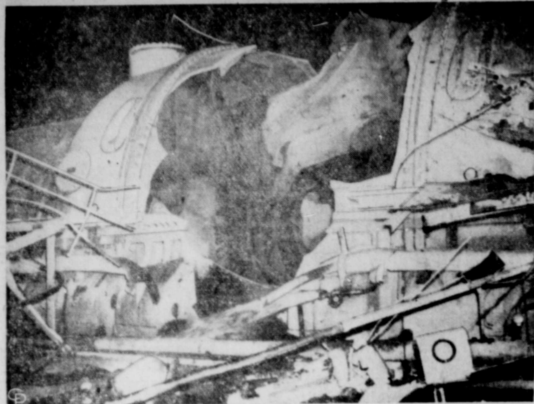
HERE IS PART of the estimated $10,000,000 damage following explosion in a six-story-high turbine electric generator of Commonwealth Edison company in Stickney, Ill., just outside of Chicago. The blast killed two men, injured five. (International Soundphoto)
