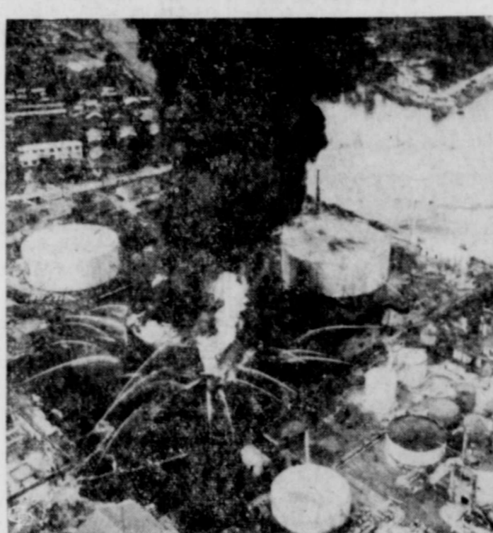
JAPANESE FIREMEN battled 30 hours to bring this petroleum fire under control in Yokkai City. Fire broke out in one tank of the Daikyo Petroleum company, then spread to three other tanks. Damage was estimated at nearly $3,000,000. Citizens had to be evacuated. (International Soundphoto)
