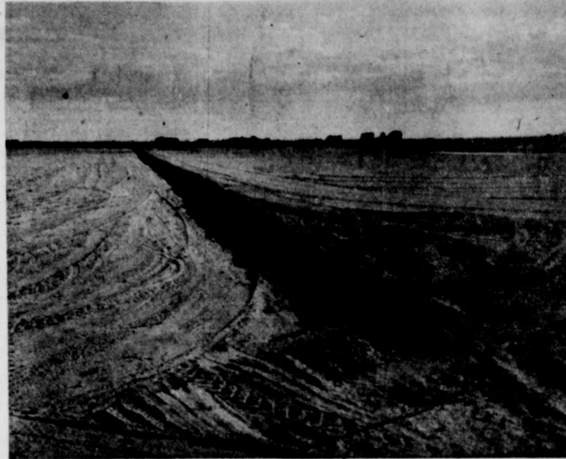
RESULTS of bench-leveling operations on the Paul Robinson farm southwest of Lake Arthur are shown in this photo. Robinson used his own equipment in working this part of his 320-acre farm.
