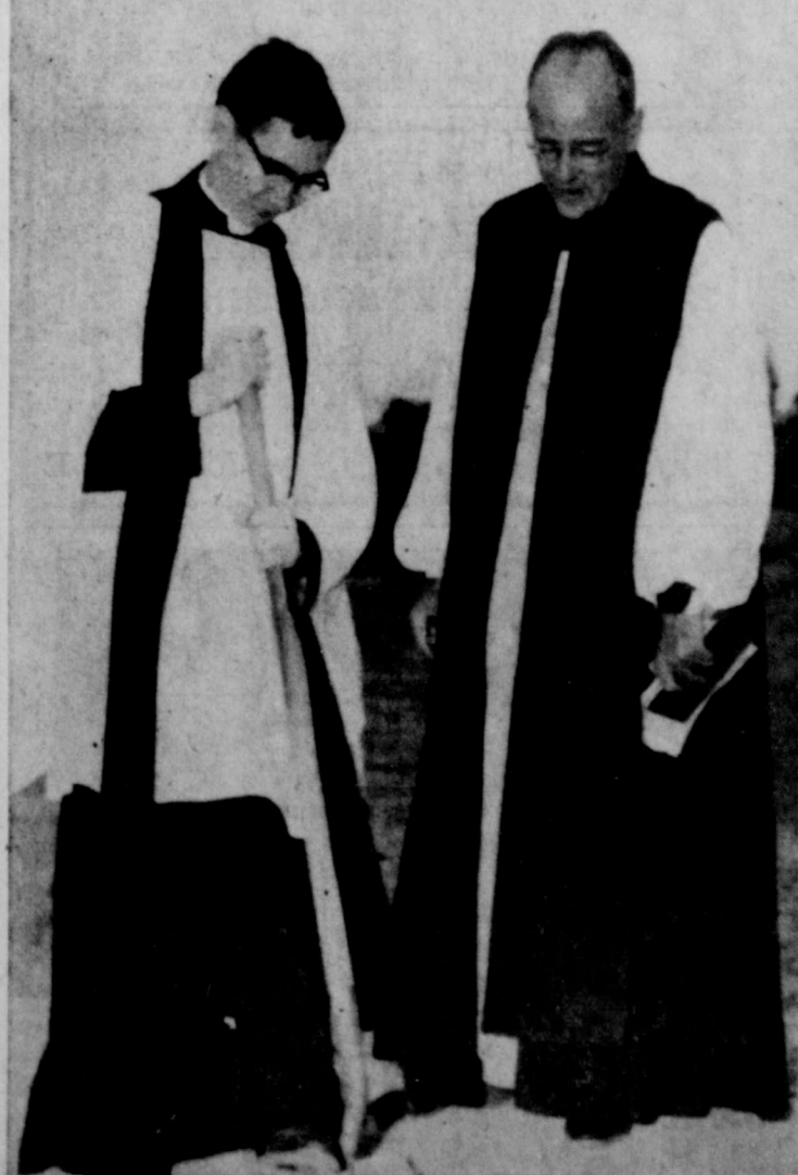
GROUND for new Artesia Episcopal church on which construction is to start this week at Tenth and Bullock was broken during ceremonies yesterday by pastor Rev. Milton A. Rohane (left) and Rt. Rev. C. J. Kinsolving, bishop coadjutor of New Mexico. (Advocate Photo)
