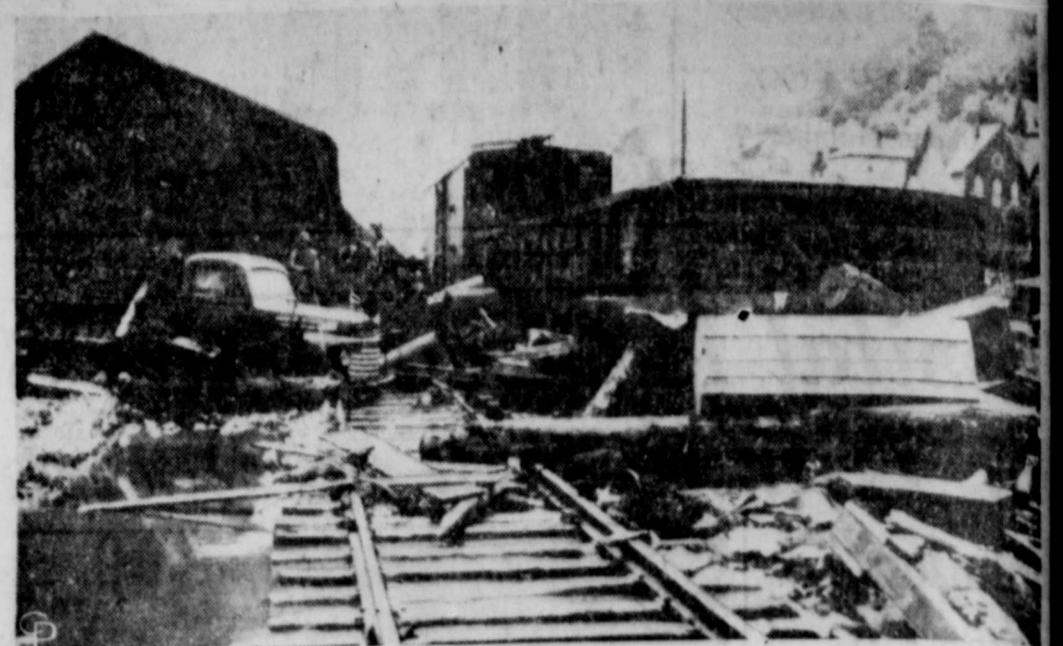
FLOOD WATER and debris litter Richwood, W. Va., as a flash flood recedes. Half the town of 5,500 was inundated, causing estimated $2,000,000 damage. Railroad is B.&O. (International Soundphoto)
