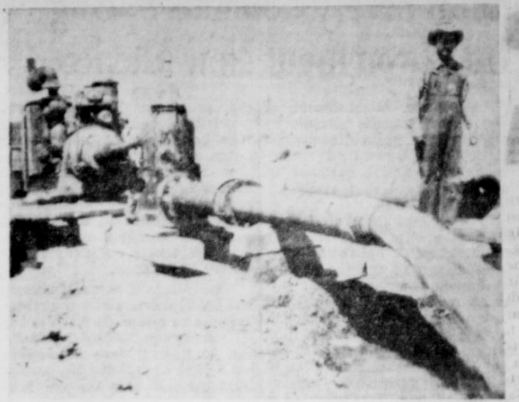
NEW WELL on farm of Mrs. G. R. Pate near Lake Arthur has recently been completed. Well pumps 1,000 gallons a minute with an 80-foot lift...
