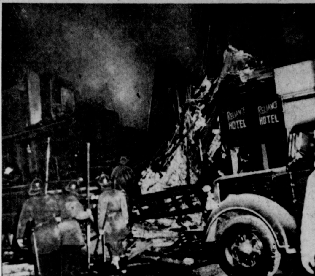
FIREMEN BATTLE a night time hotel fire in Chicago in which at least one fireman was killed and 22 others were injured when the roof, front and side walls collapsed. Several firemen were buried in the debris and feared dead.
