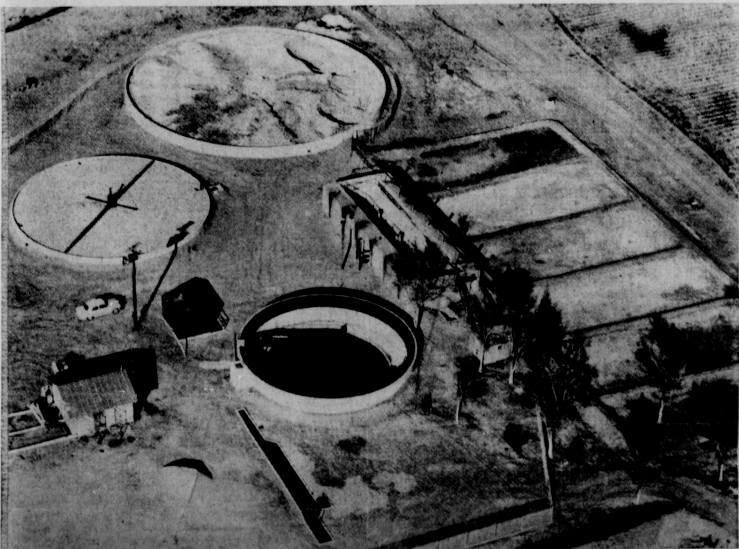
AERIAL PHOTO shows size of big new Artesia disposal plant. All equipment and structures are new except re-
