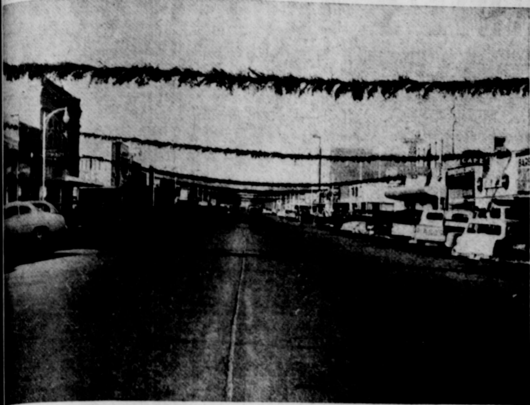
MAIN STREET is ready for Christmas with these gay decorations erected Saturday by workmen from four utility companies and the city's electrical contractors. Evergreen roping is new to Artesia Yuletide motif and exceptional in the Southwest. (Advocate Photo)
