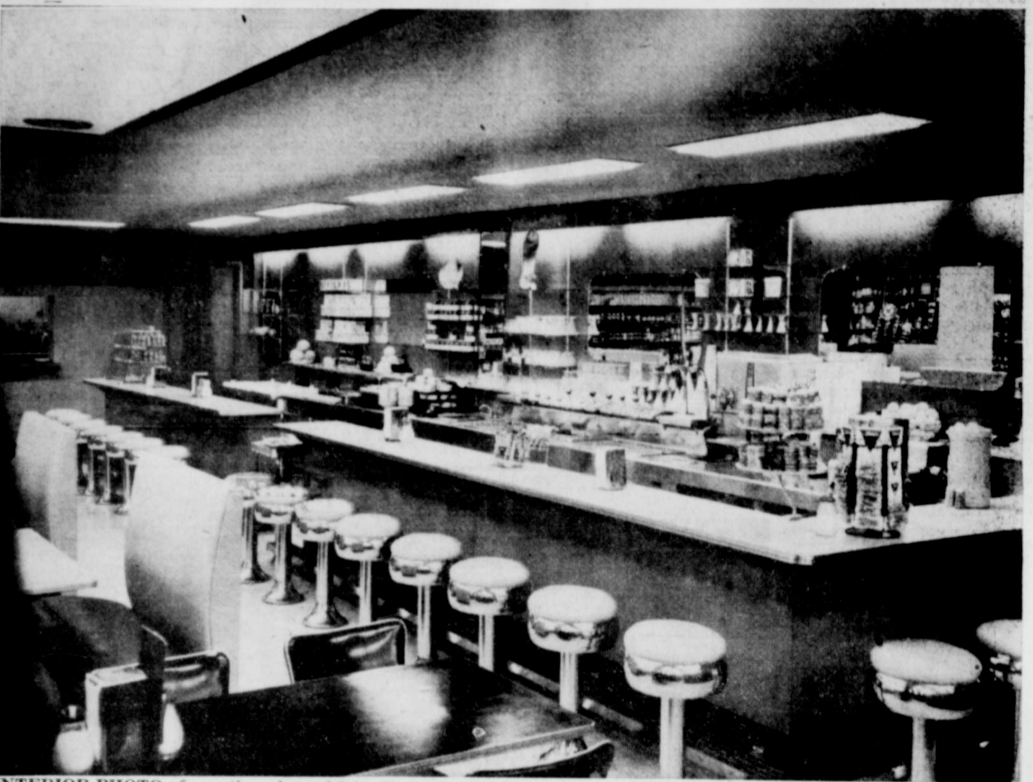
INTERIOR PHOTO of greatly enlarged Irby Drug Store indicates openness which addition of 360 square feet of floor space have added. Irby is holding grand opening of remodelled, enlarged drug store today. Complete new fountain and lunch facilities have been added, and seating capacity doubled. Store is completely departmentalized for group arrangement of related products. (Photo by Gable)
