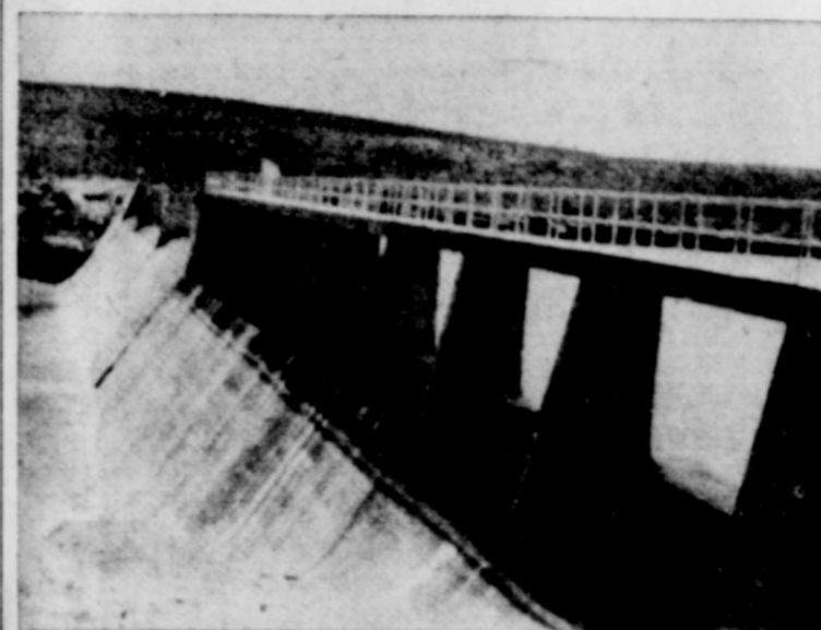
THIS IS THE dam which will once again run west of Hope, thanks to a $75,000 appropriation authorized Saturday by the state finance board. This photo was taken shortly after completion of the dam in 1941, before it filled with silt, becoming useless.
