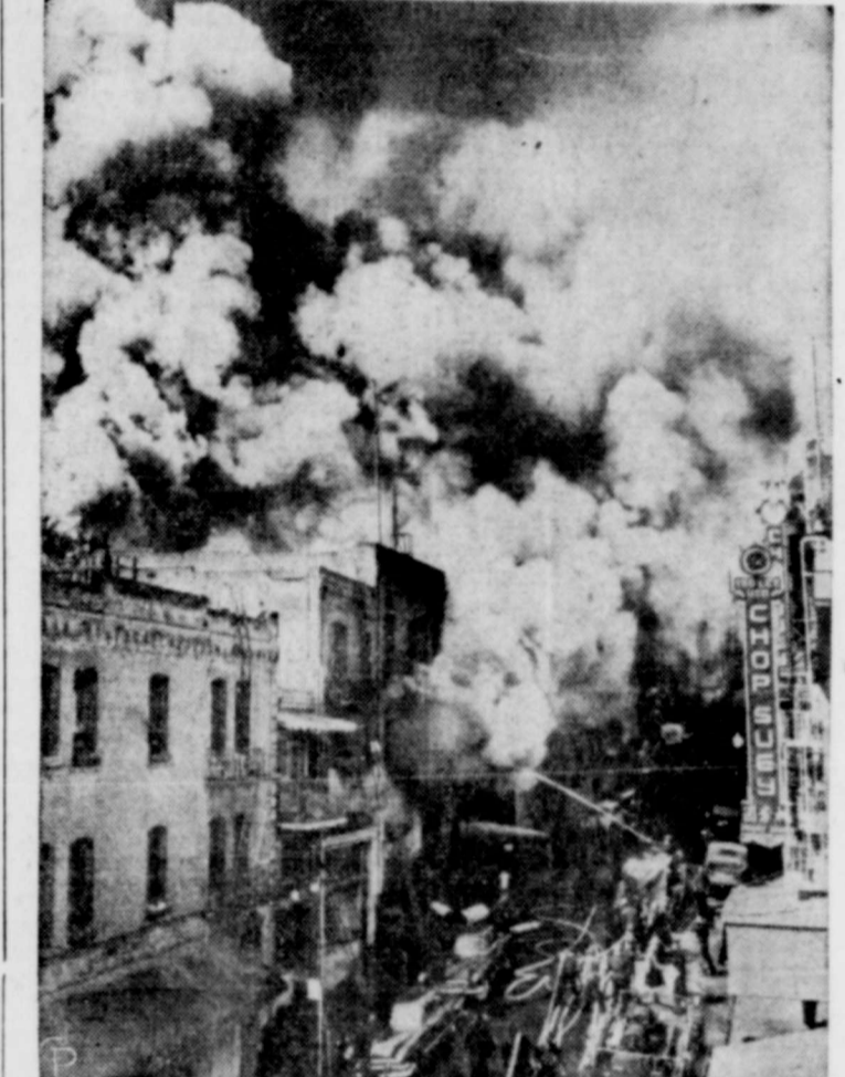
SMOKE BLOTS OUT the sky over Chinatown in San Francisco as a four-alarm fire rages following an explosion in a plumbing shop. Nearly all fire fighting equipment in the downtown area answered the call. Five persons were injured, three seriously. (International Soundphoto)
