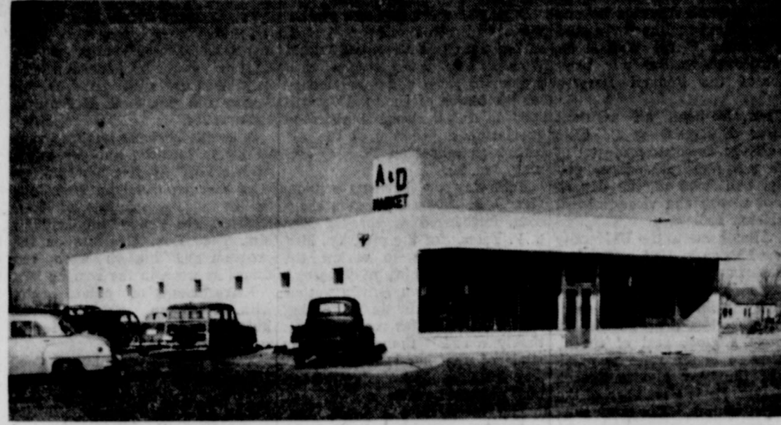
EXTERIOR PHOTO of new A&D Grocery and Market in the 600 block of N. First street give a hint of the big parking area, which extends all the way around the building. Little tower with company trademark on it readily identifies building for customers. New building is 100 by 50 feet, more than four times as large as the building occupied by A&D when the Kennedys bought it six years ago.
