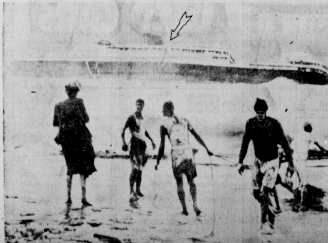
ARROW INDICATES big crack amidships in the French liner Champollion as she wallows helplessly in pounding waves several hundred yards off Lebanon coast. Liner struck a reef. (International Radiophoto)
