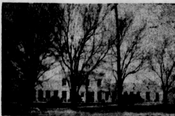
VIEW OF ANNEX
