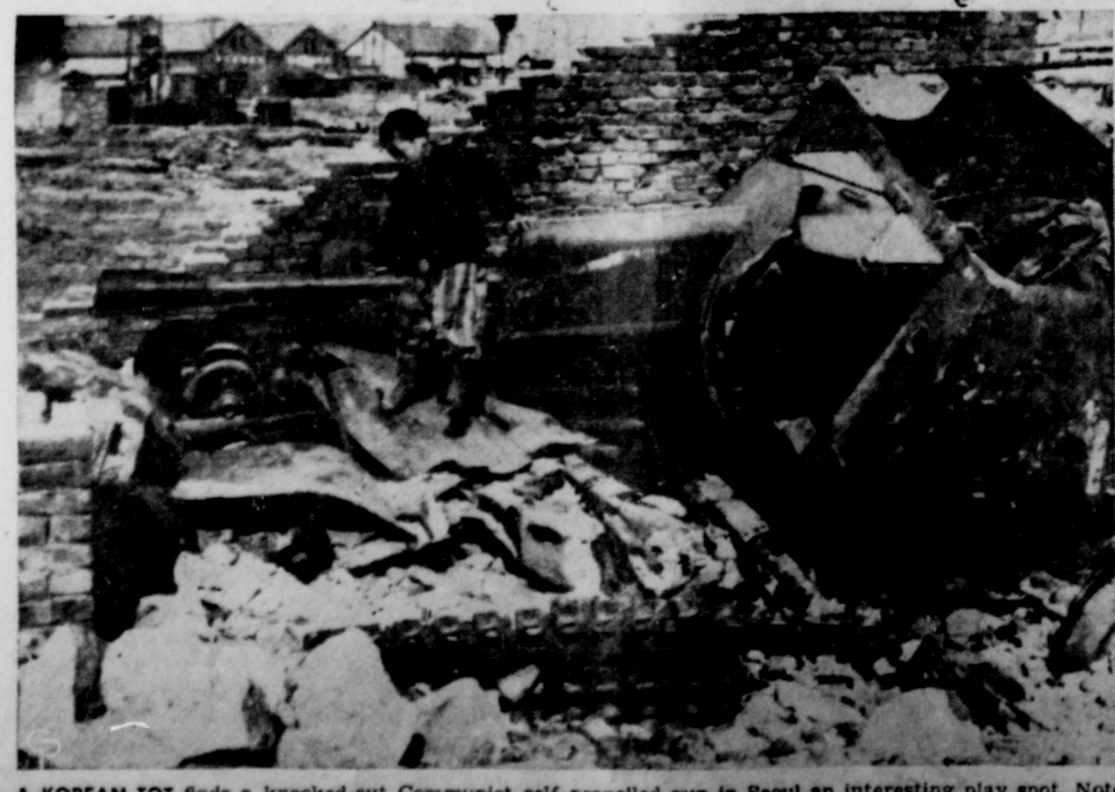
A KOREAN TOT finds a knocked-out Communist self-propelled gun in Seoul an interesting play spot. Note the war damage to buildings in the scene. Defense photo.
