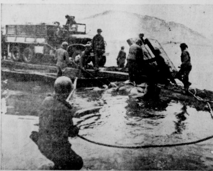
A 2 1/2-TON TRUCK is unloaded from a ferry built of assault boats for crossing the Han river near Seoul, Korea. It was pushed across flooded Han by outboard motor. Defense photo. (International Soundphoto)
