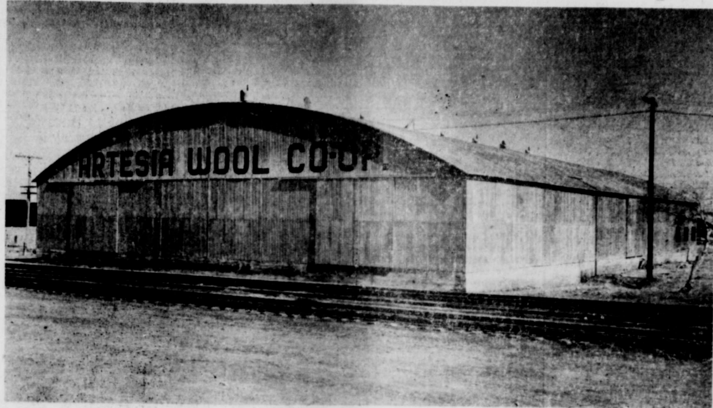
Here is the huge, 100x160-foot corrugated steel, pre-fabricated warehouse building on Mosley Avenue just east of the Santa Fe tracks, which has just been completed for the newly-organized Artesia Wool Co-operative, the opening of which was announced this week by Bryan Runyan, president.
