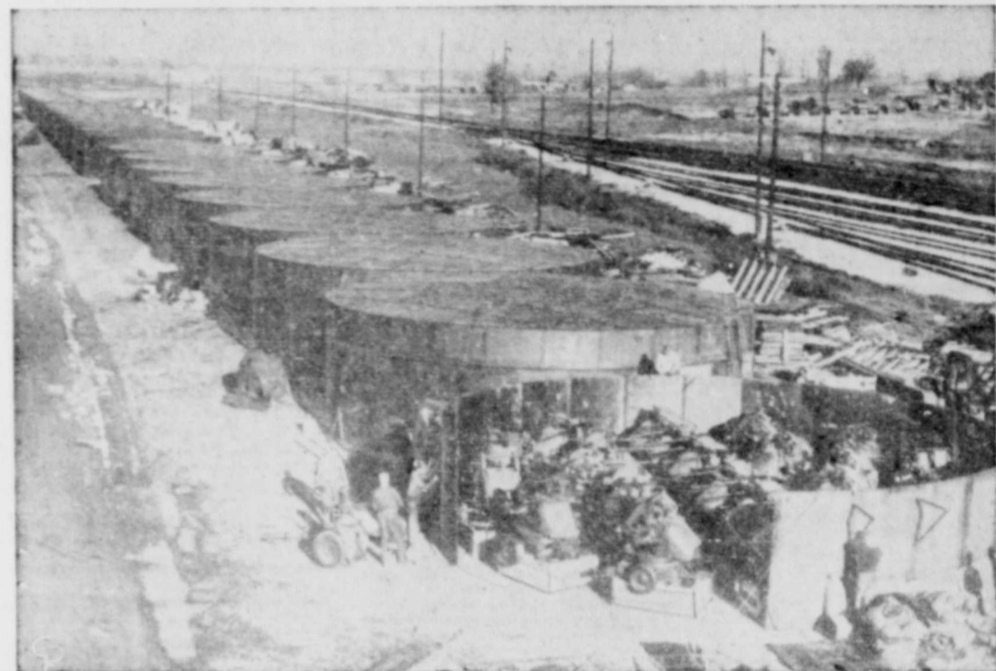
A long line of material containers at Chambersburg, Pa. Supply of gun mounts is stored in foreground. THANKS TO PLANNING and ingenuity, the U. S. is better prepared today than before Pearl Harbor. Eight ordnance depots are equipped with steel storage containers full of combat vehicles of various kinds, many of which are now coming out of their "mothballs." An intricate system of air conditioning prevents rust, preserves Grade "A" condition. Storage costs only fraction of replacement. (International)
