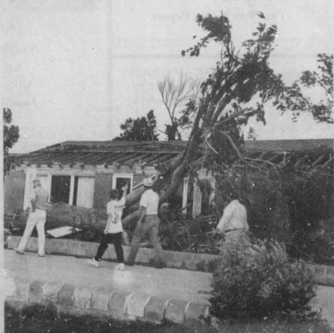
TORNADO TAKES SWIPE AT BILL JIM ST. CLAIR HOME--Just west of the J. D. Cage home near Muleshoe on Highway 70, is the home of Bill Jim and Marlene St. Clair. A tornado moved from the southeast to the northwest, until after it struck the St. Clair home, then veered to the northeast. (Journal Photo)
