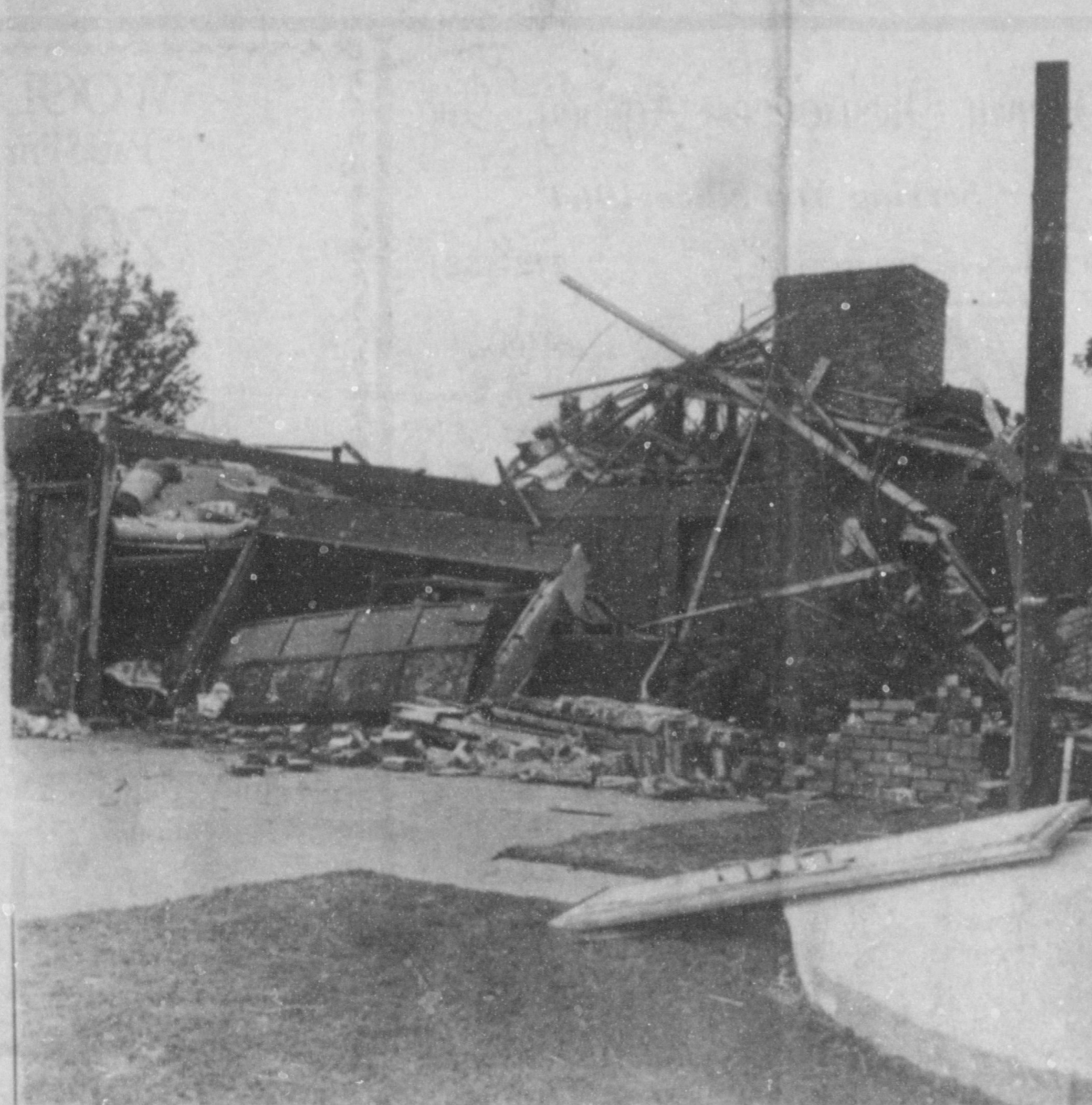
WHAT WAS LEFT OF THE BACK OF THE CAGE HOME--Tangled wreckage, mangled vehicles and twisted wire was virtually all that was left of the back of the J. D. Cage home late Saturday afternoon when a large tornado whirled through it. The Cage's were at their ranch with guests, and were not injured in the tornado. (Journal Photo)
