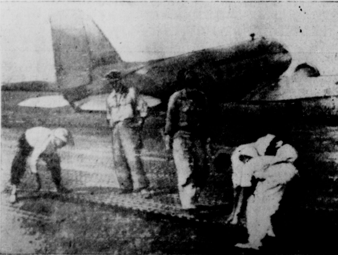
KOREAN LABORERS lay a prefabricated airstrip in South Korea, with an American overseeing the job. Lack of such facilities has hampered Air Force operations in the war. (International via Army Radio)
