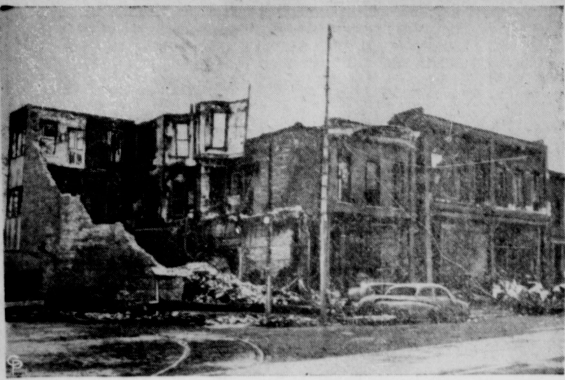
ALMOST DESTROYED is this block of Chicago buildings following the explosion of a tank-truck, carrying 8,000 gallons of gasoline, after it was hit by a streetcar. Fifty families were made homeless and four children reported missing. Cars parked in the street were also burned. The death-toll of the trolley disaster was placed at 33 persons, with 50 injured. Cause of the crash is being investigated. (International Soundphoto)
