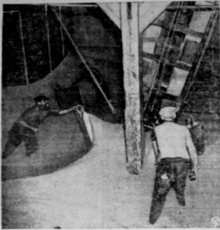
COPING WITH THE SHORTAGE of grain storage facilities, the United States has decided to use a fleet of twelve ships anchored in the Hudson River for storing grain from the bumper crop now being harvested. Here, workers at the Claremont Terminal in Jersey City, N. J., pour surplus wheat into the Benjamin Hawkins. The Government has also offered long-term low-income loans to farmers as an inducement in helping them build their own storage bins. (International Sound/photo)
