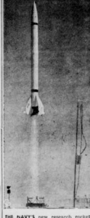
THE NAVY'S new research rocket "Vicking" is shown as it roars skyward in second successful flight at the White Sands Proving Ground Las Cruces, N M. The missile reached an altitude of 33 miles, carried four cameras, and radioed back o earth some forty different kinds of scientific information during the ive minute flight. (International)
