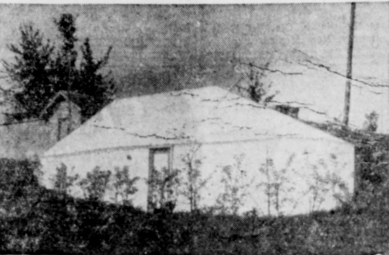
Concrete Front Large Vegetable Cellar
