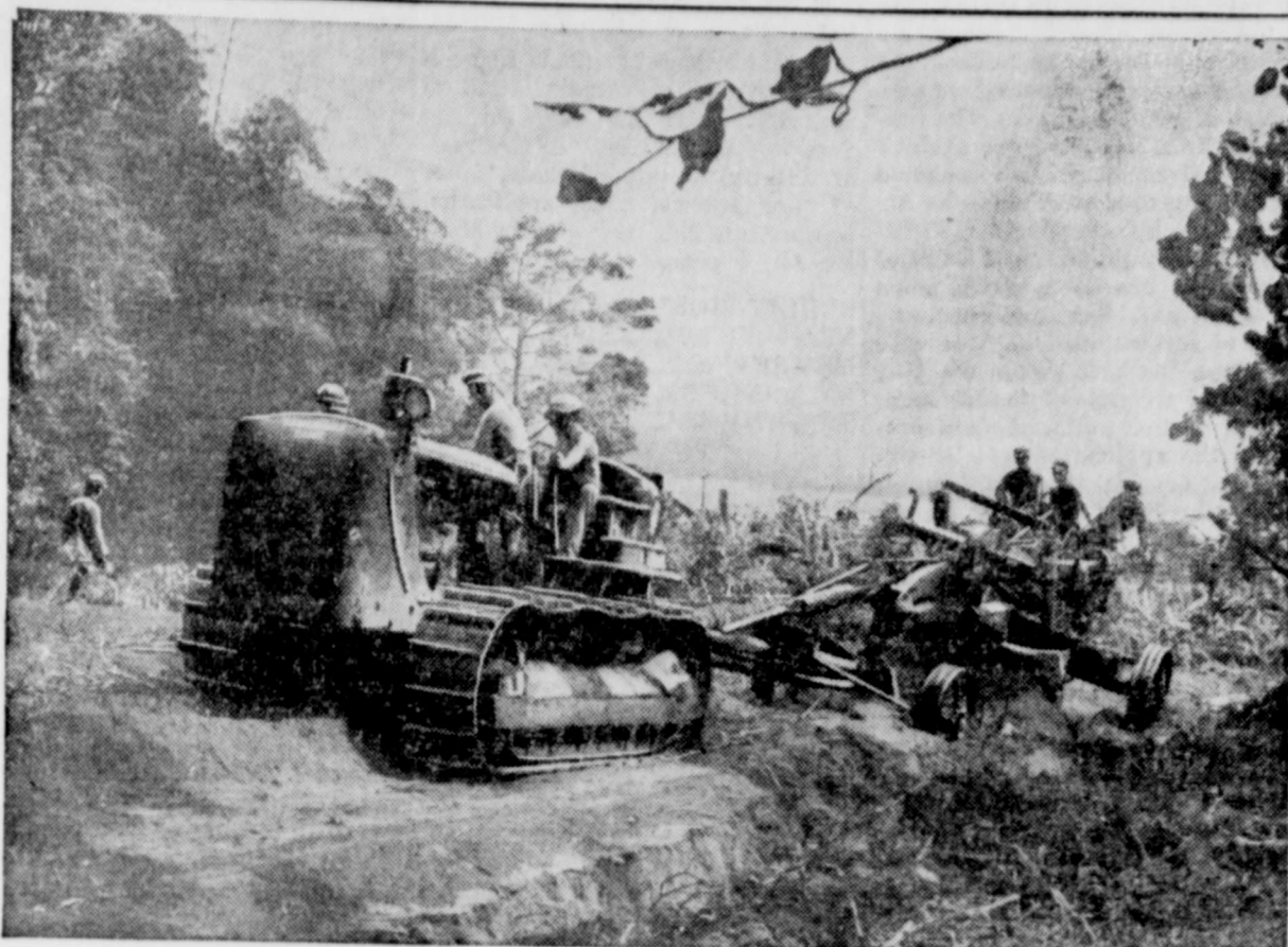
That is the name our engineers call this tractor just as tank men name their tanks and fliers their ships. Starting from scratch these men are driving this road through the jungle in the Sansapor Area of Dutch New Guinea. The tractor is hauling a road grader along a clearing. Your War Bond purchases assure our fighting men of the best of equipment and here you see some of it at work.
