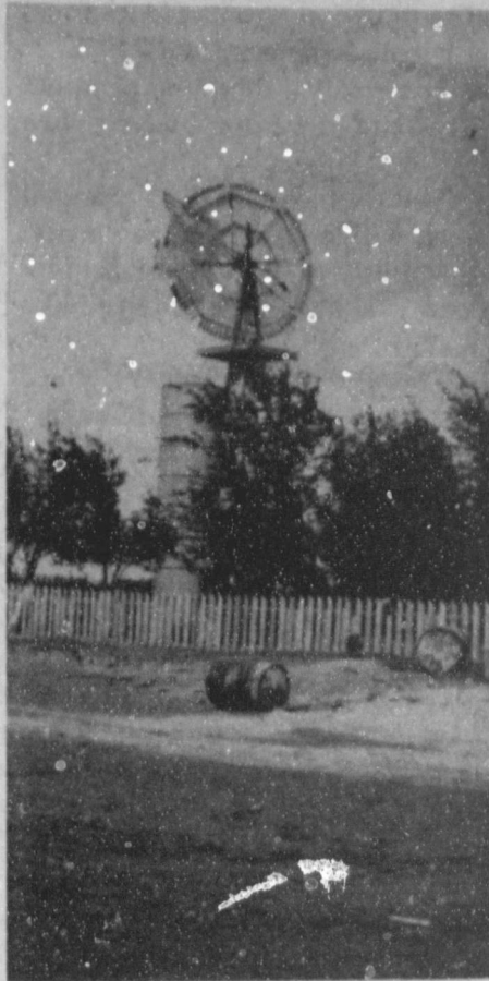
WATER SUPPLY ---Muleshoe's first source of water was the old windmill and overhead storage tank.
