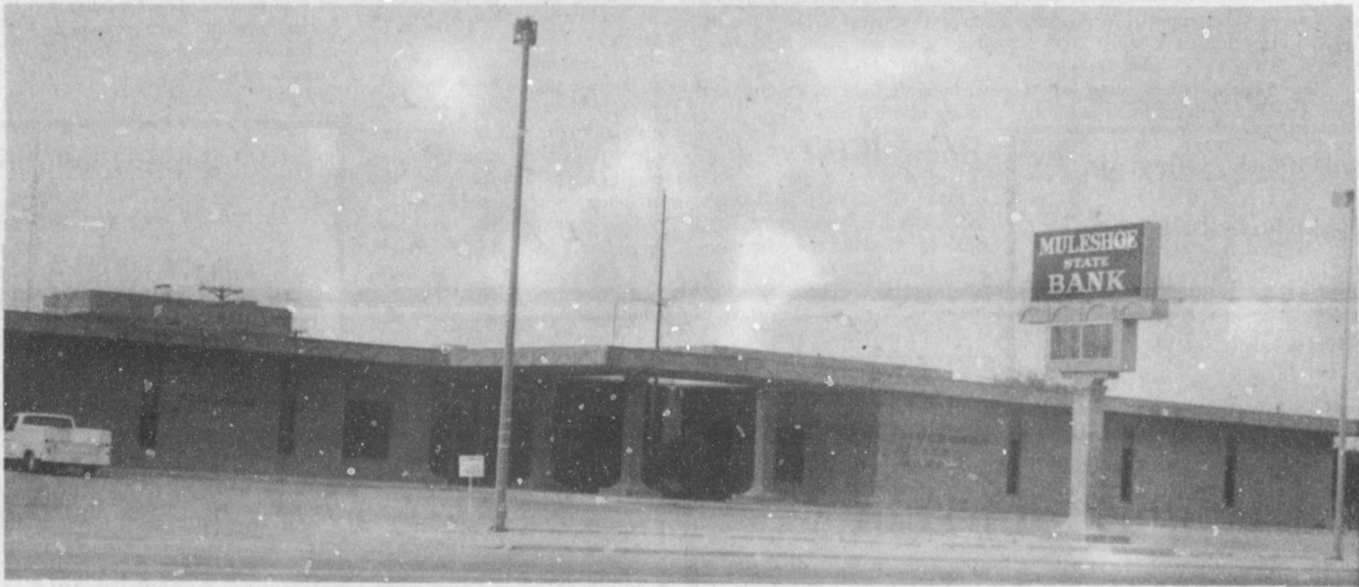
The New Muleshoe State Bank
