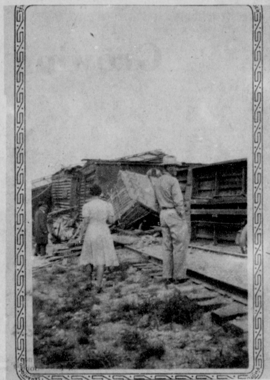
LOOKING OVER THE DAMAGE--These unidentified sightseers take a look at the damage when a freight train derailed in the 1940's between Muleshoe and Progress. (Guest Photo)
