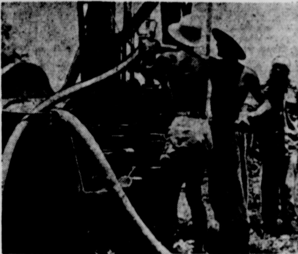
SOUND WAVES set up by the firing of a charge of dynamite 15 to 60 feet below the surface help Atlantic Refining Company exploratory crews locate likely oil-bearing formations in Cuba's Santa Clara Province. The photograph shows the machine used to drill the hole for the dynamite charge.
