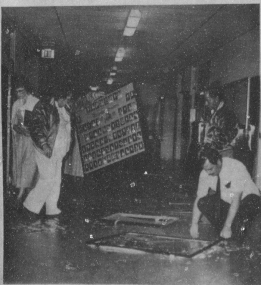
Beginning clean-up of debris
