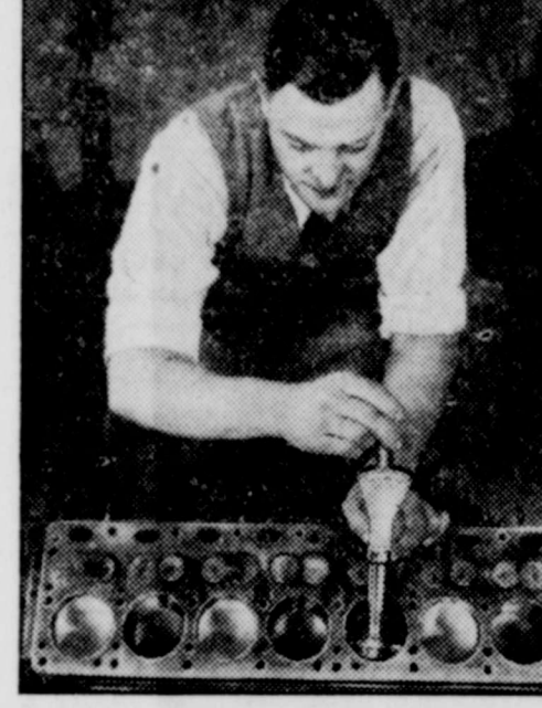
Measuring cylinder wear with a precision gauge—accurate to a hundred-thousandth of an inch!
