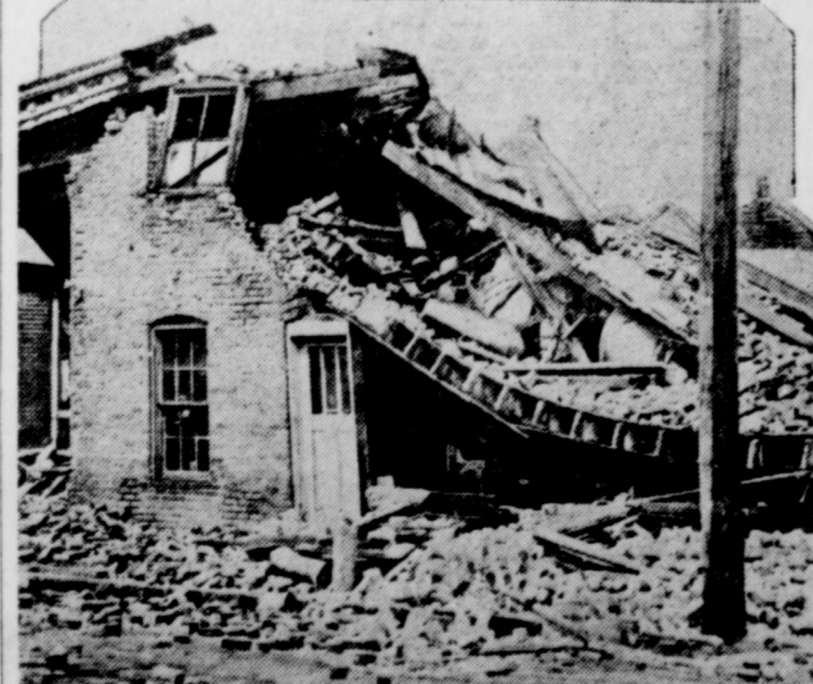
View in Dayton, Ohio, after a freak tornado struck the west side of the city, causing property damage estimated at several hundred thousand dollars and injuring a number of citizens. The high wind was accompanied by torrential rainfall and hail.
