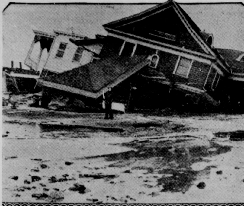
Wreckage of the Hinkman house, in Seabright, N. J., after it was demolished by the terrific gale which swept along the Atlantic seaboard. The heavy surf driven by the high winds washed away shore foundations at many resorts. Mountainous waves tore boardwalks to pieces and scores of homes were blown from their bases.
