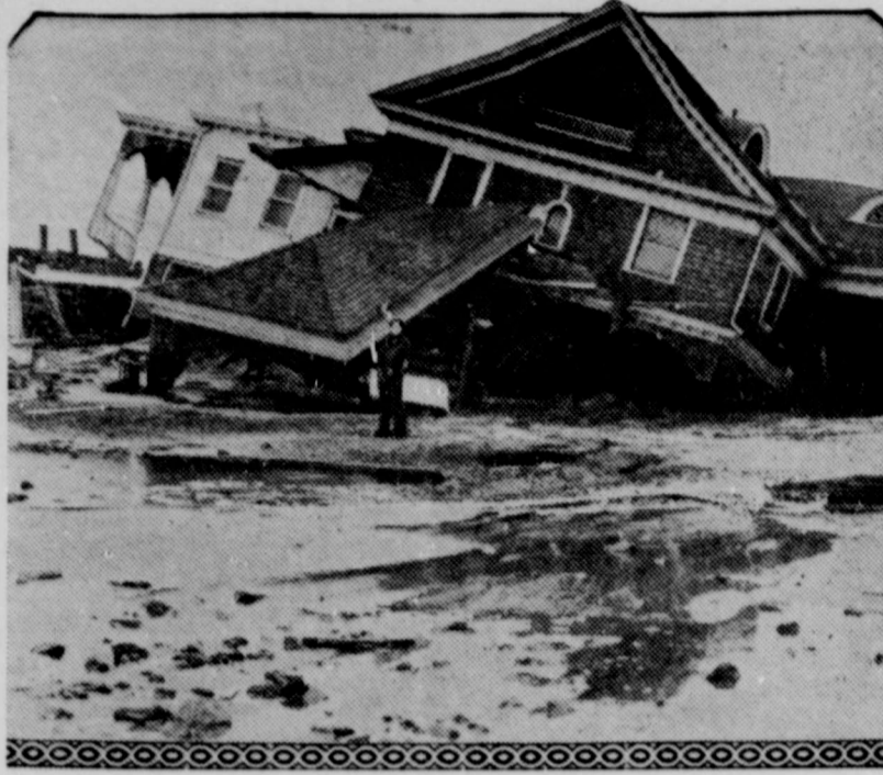
Wreckage of the Hinkman house, in Seabright, N. J., after it was demolished by the terrific gale which swept along the Atlantic seaboard. The heavy surf driven by the high winds washed away shore foundations at many resorts. Mountainous waves tore boardwalks to pieces and scores of homes were blown from their bases.
