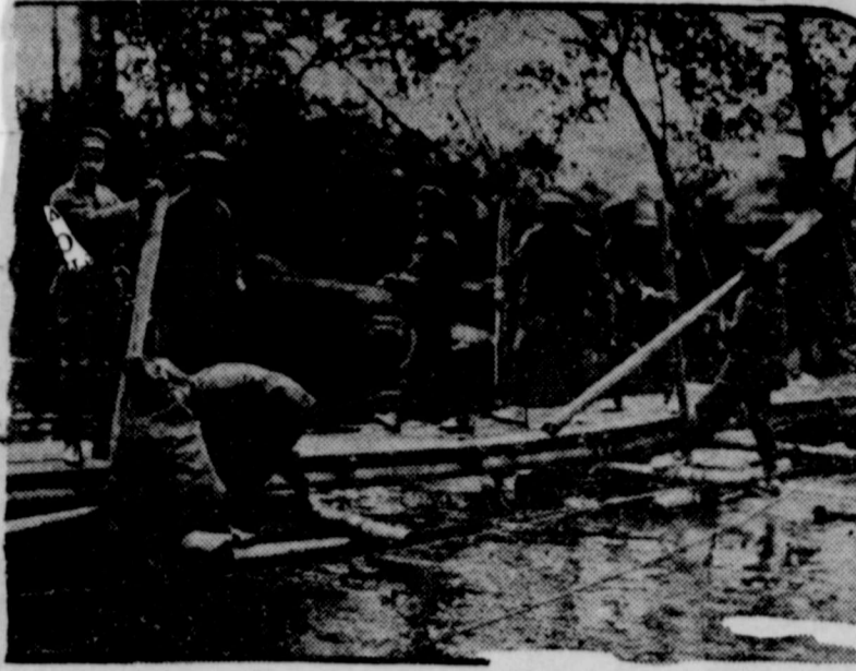
Dispatches from Para, Brazil, say Colombian naval vessels have used up the Amazon carrying munitions and 1,000 troops to the Letitia region over the possession of which Colombia is disputing with Peru. The picture shows Colombian soldiers building a pontoon bridge under ar conditions.
