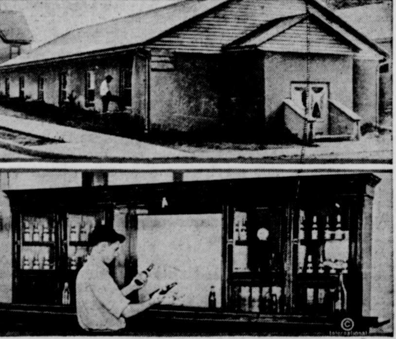
The little abandoned church seen above is on a quiet street in Clifton, N. J. Recently prohibition agents noticed it was drawing an astonishing number of "worshippers," and on investigation they discovered the fully furnished bar shown in the lower part of the picture.
