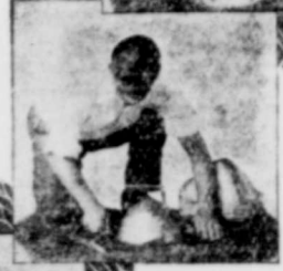
4—Tamp Soil Around Edge of Setter
