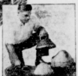
4—Tamp Soil Around Edge of Setter
