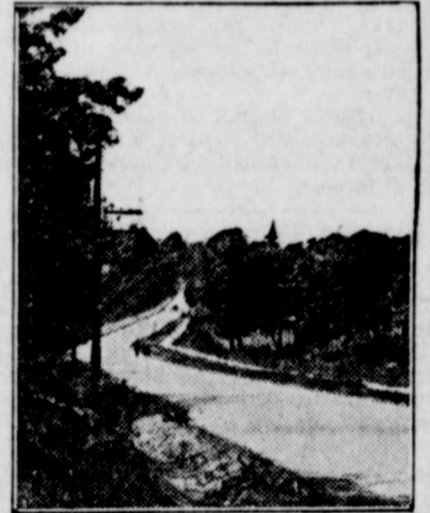
A Completed 20-Foot Concrete Road.
