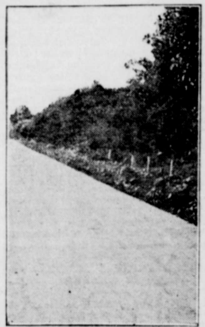
A Federal-Aid Concrete Road in Minnesota.
